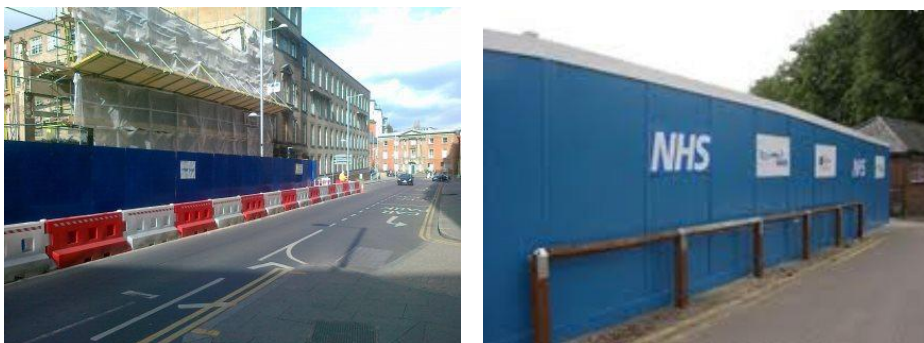
Above Left: Bowmer & Kirkland, Nottingham Centre, Right: Interserve, Maidenhead.
