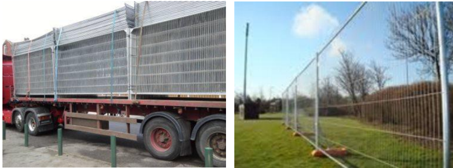
Above Left: 240 anti-climb panels (only) on an artic, right: anti-climb panels erected.
